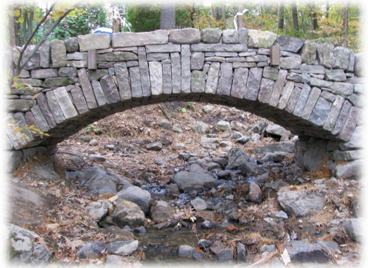
A dry-laid footbridge in Landon Bay, Ontario.
